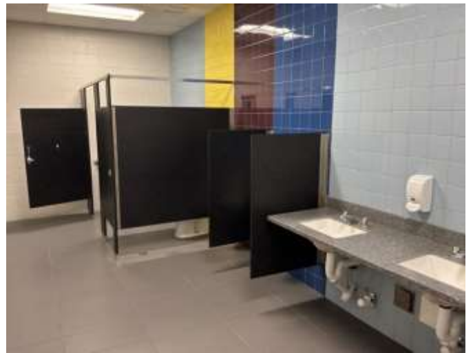
28 - RENOVATED RESTROOM OVERVIEW
