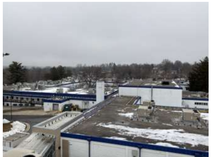
6 - MAIN ROOF OVERVIEW
