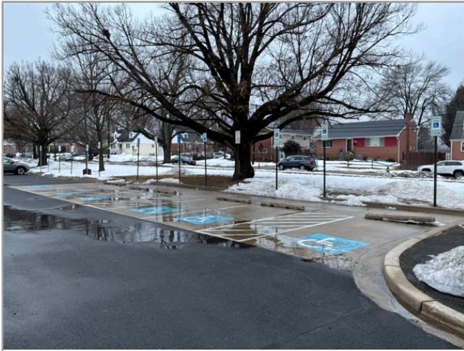
OVERVIEW OF ACCESSIBLE PARKING AREA
