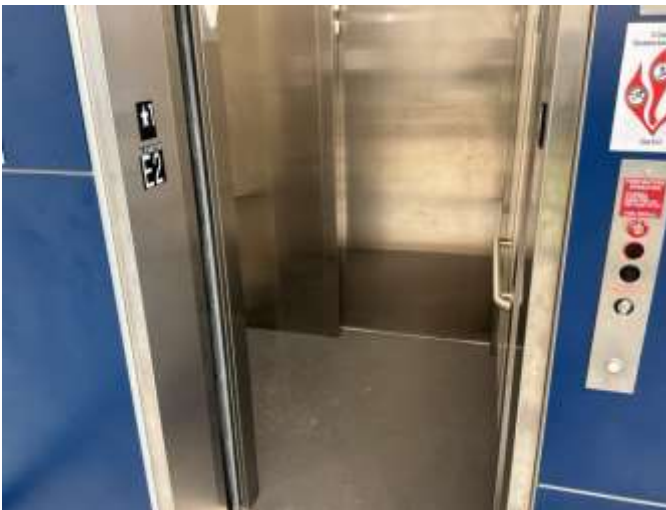
33 - ELEVATOR CAB FINISHES
