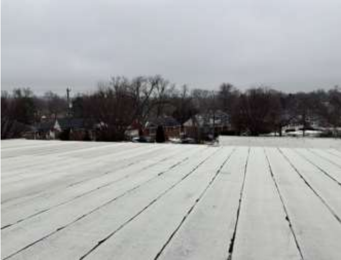
7 - SECONDARY ROOF OVERVIEW
